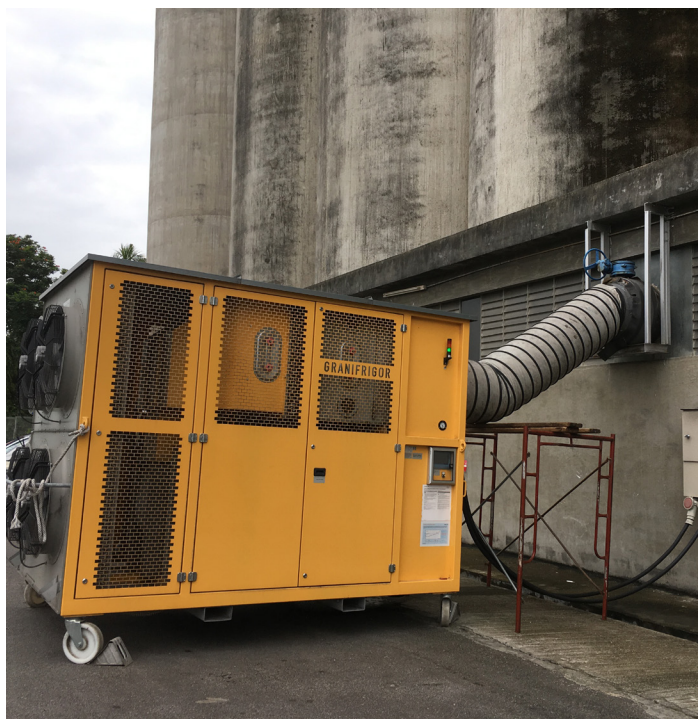
Figure 10. Grain chiller used to insert cooler air into each of the storage silos that had the grain chilling treatment ( www.frigortec.com ).
